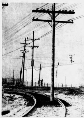
A TRAIN would have difficulty getting around this pole on a railroad spur in Waukena, a Milwaukie, Wis., suburb. The pole was here first and the track extension for a new industry was built around it.
