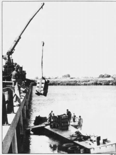
A crane removes boxes of the hazardous cargo from the submerged truck.
