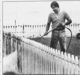
Having a blast Dave Powell seems to be having a blast using a high pressure water sprayer to remove old paint Friday
