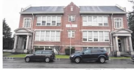
▲ If a Tacoma schools bond passes in February, the facade of Oakland High, built in 1902 as an elementary school, would be saved and the interior gutted. Photo taken on Wednesday, Jan. 22, 2020.
