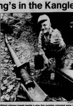
Wilford Johnson kneels beside a pipe that supplies untreated water to the town of Kangley.
